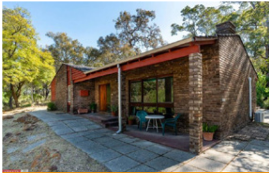
Figure 13 - Bailey Road, Glen Forrest Source: CoreLogic
