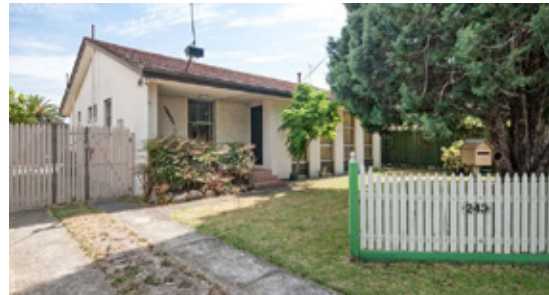
243 Cheltenham Road, Keysborough Source: realestate.com.au
