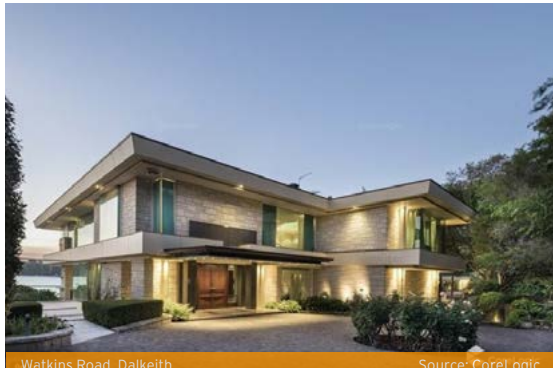
Watkins Road, Dalkeith Source: CoreLogic
