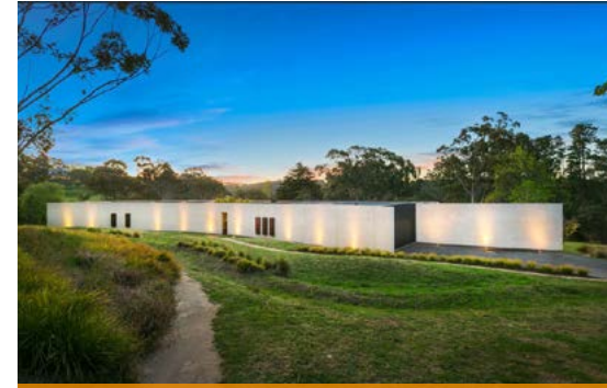
14 Williams Road Heathfield Source: realestate.com.au
